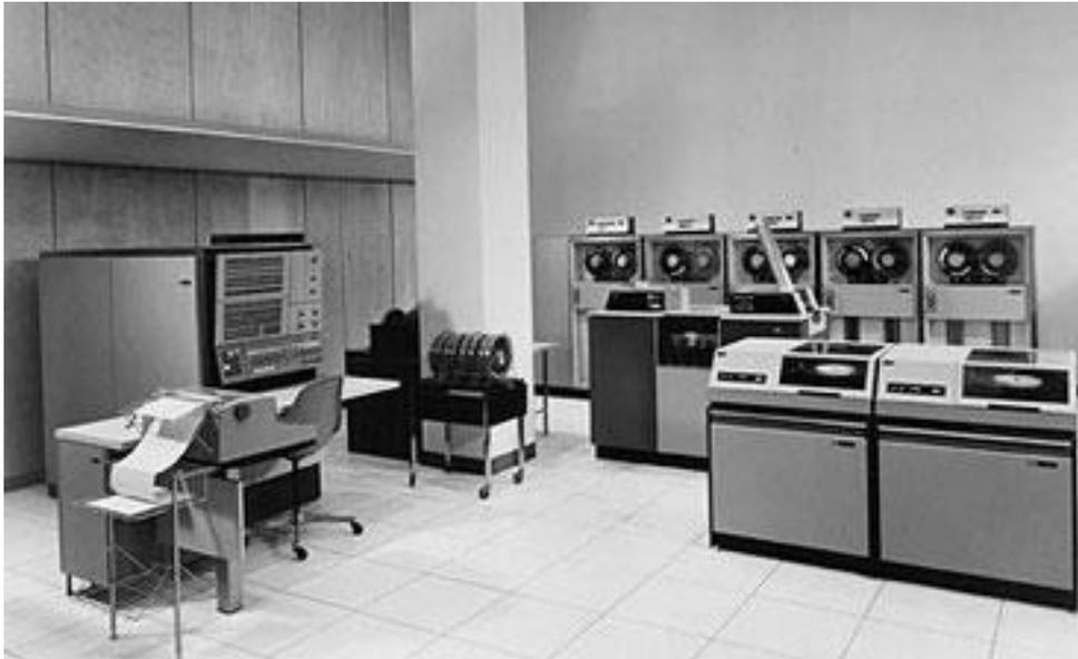
Above, the S/360 central processing unit is on the left against the wall, with the typewriter-like printer in the foreground on the left. Five tape drives are on the right in the rear, with two disk storage units in the foreground on the right; in between these is the card punch/reader. Collectively, when coupled with an operating system, these constituted the mainframe environment, although in today's parlance, the word mainframe tends to refer only to the central processing unit.
